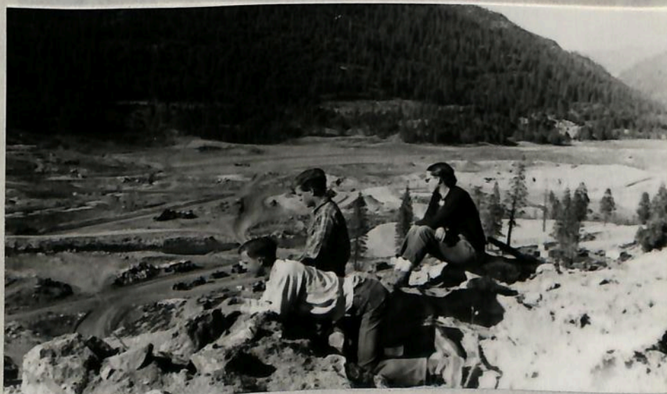
Photo 12. Beardsley Dam site; excavation almost complete. View is up-stream from above the east abuttment. Jim, Jon and Arlene. 1955.
