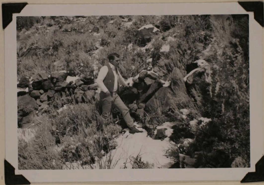
Photo 2 - Close-up of wall shown in Photo 1.
