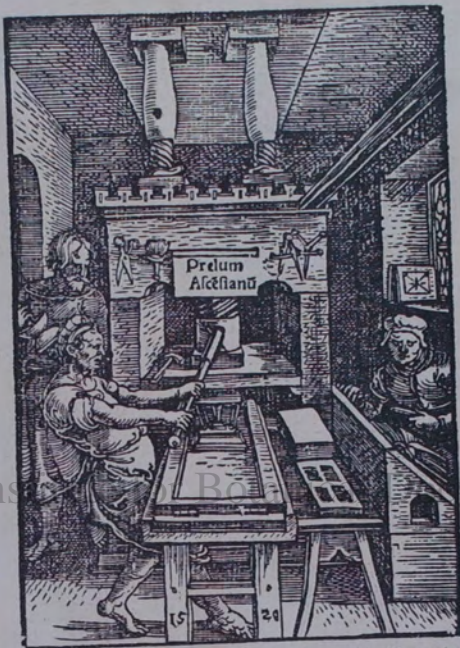
16TH CENTURY PRINTING PRESS.—This illustration from a book printed by Jodocus Badius, Paris, 1522, shows an early wooden hand press. It will be noticed that the upper part was fixed to the ceiling.
