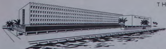
NEW HERALD BUILDING NOW UNDER CONSTRUCTION
