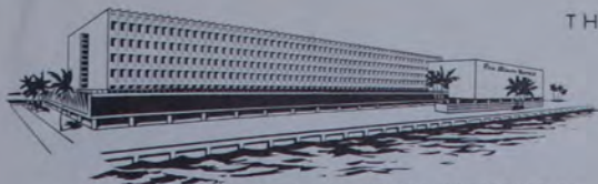
NEW HERALD BUILDING NOW UNDER CONSTRUCTION
